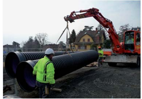
Transport des tubes PE, diam. 850
